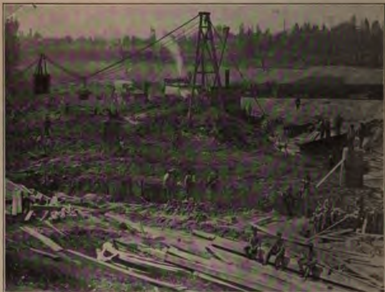
Cableway Excavator Digging a Sewer Trench.
